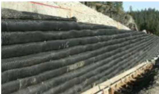
Figure 1: Typical wrapped face MSE walls
